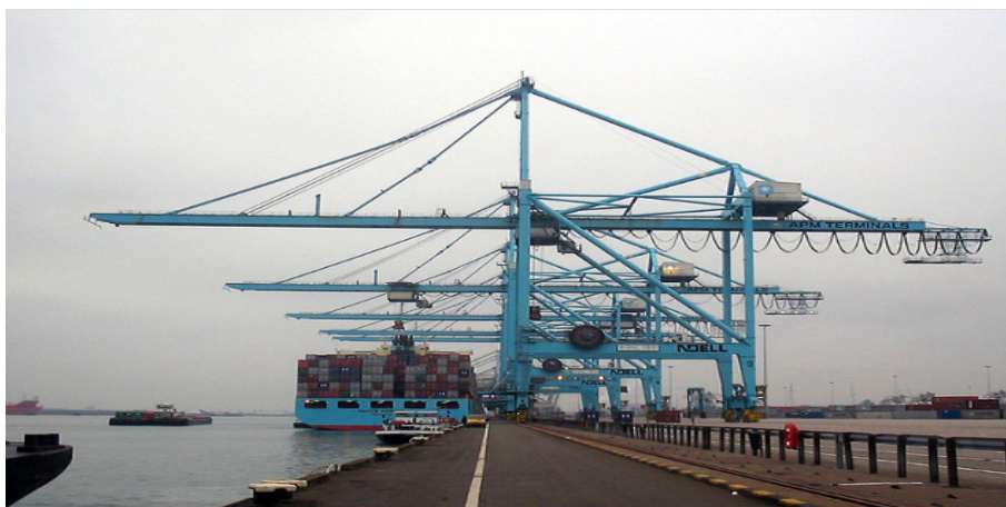
FIGURE 1.3: Gantry Cranes at a seaport
